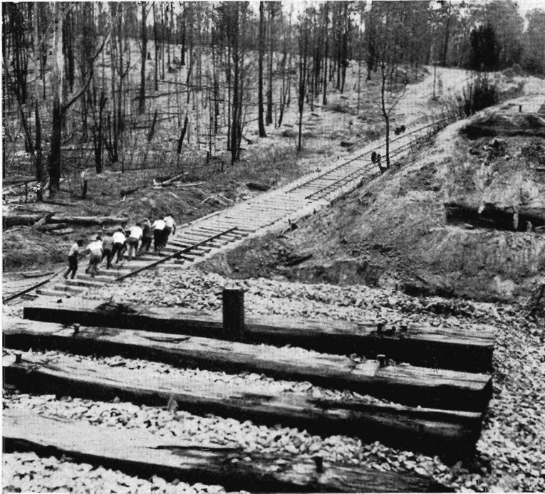
Laying track for a deviation. Grade is 1 in 20.
