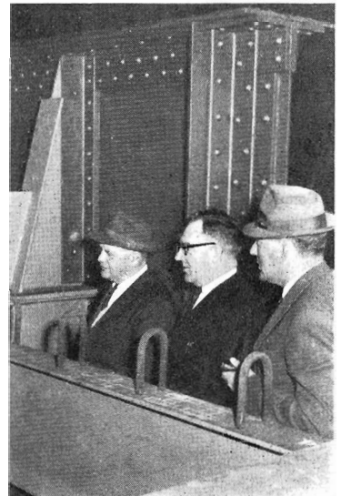
At Newport Workshops, Messrs G. F. Brown, Deputy Chairman of Commissioners, (left), S. F. Keane, Assistant Chief Mechanical Engineer, and D. D. Wade, Acting Chief Civil Engineer (right), inspect the fabrication of steel girders for the Mordialloc Bridge.
