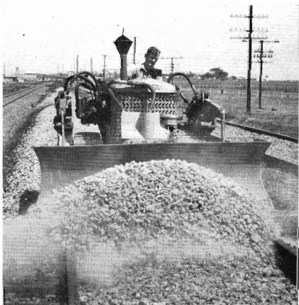
Ballast is distributed with tractor and spreader.
