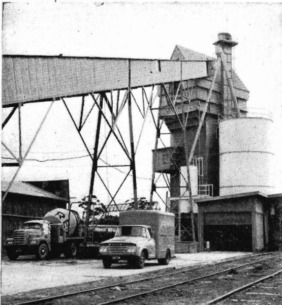
Arden Street plant of Ready Mixed Concrete Pty. Ltd.
