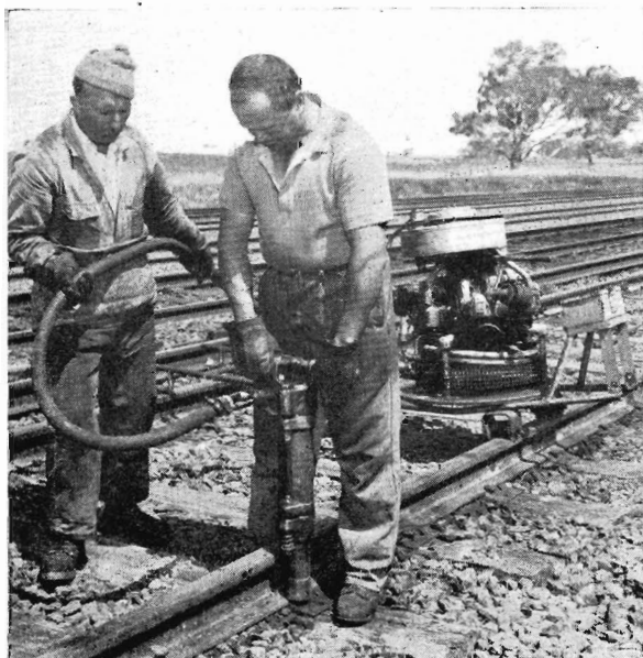
Dogspikes holding the new rail are driven with pneumatic spike hammer.
