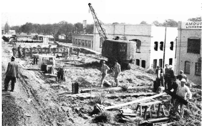
Constructing new platform at Richmond.
