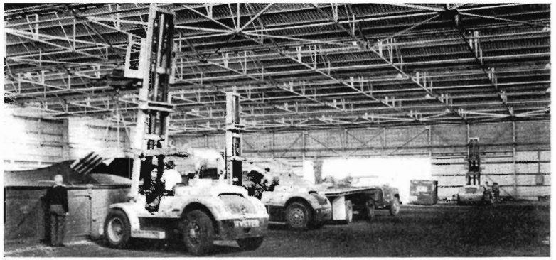
A heavy fork lift truck works in the spacious weather-protected South Dynon goods shed where goods are transferred between rail and road vehicles.
