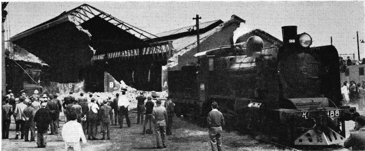
K 188 brings down the front wall of North Melbourne Locomotive Depot.
