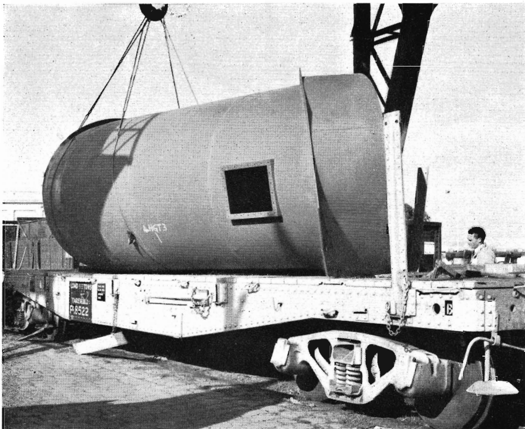
UNUSUAL LOAD : Railways play a vital part in hauling large and massive equipment needed for power stations. A hot-air duct is being loaded at Melbourne Goods for the State Electricity Commission's huge new power station at Hazelwood.
