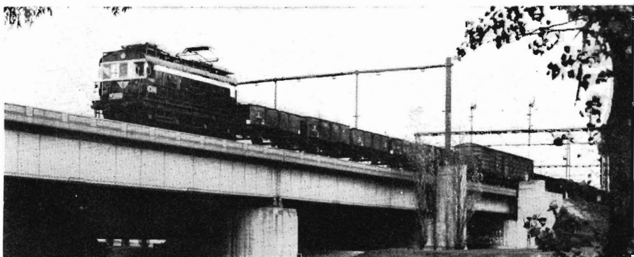
BLUE AND GOLD: This E class suburban goods electric locomotive, shown hauling a train across the Cremorne Bridge, South Yarra, is the first of the class to be re-painted blue and gold – the standard V.R. livery. The original colour was black.
