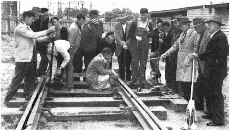
Some of the 26 repairers who are attending the training school for gangers at Dandenong are shown receiving instruction from Road Foreman S. Hall (third from right).
