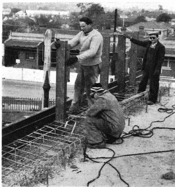
Members of Special Works gang are concreting the road surface of overpass. When completed, this overpass will eliminate the busiest part of the metropolitan area. Workmen are erecting protective fencing.
